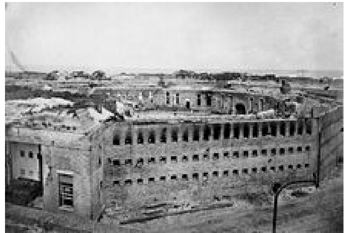
Aug 23, 1864, Damage to the Citadel
